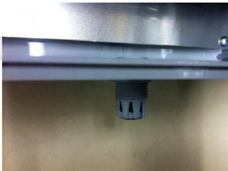
8. Attach the nut on top of the cord grip to secure the cord grip to the enclosure.
