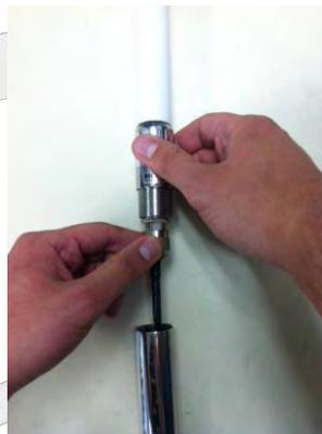
17. Wrap one of the black 3" weather tape strips around the connection of the antenna and coax cable.
