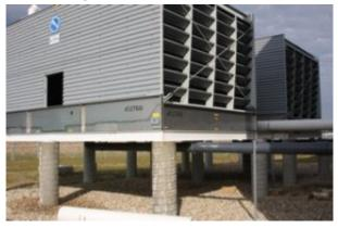
Redundant cooling towers provide heat rejection from critical IT loads.
